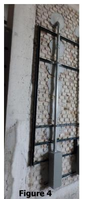
**Vertical Installation** – (Figure 4) – Vertical runs require an enclosure (pull box) be installed at the bottom of the raceway. The bottom raceway must exit through either the back or side wall of the enclosure. Vertical runs may utilize an enclosure (pull box) elsewhere within the system. The cable(s) shall enter and exit through the top and bottom of the
